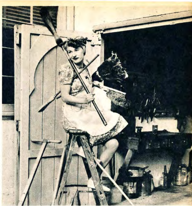
One hour later she sits wistfully surveying the exterior of the house weighing the knotty problem of "Where do I start" And How?
